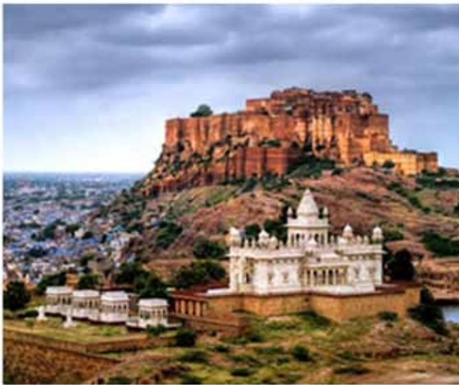
Mehrangarh Fort, Jodhpur Rajasthan, a conservation project by Ar Meenakshi Jain
